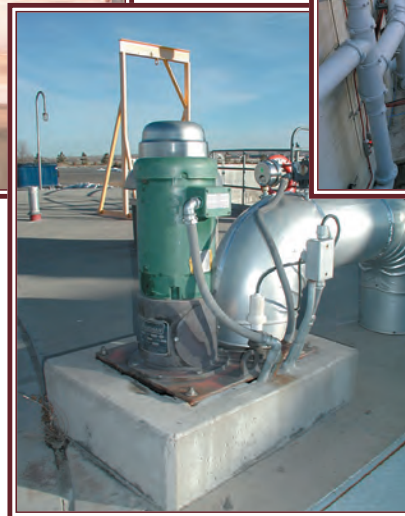
Primary Clarifier Scum
