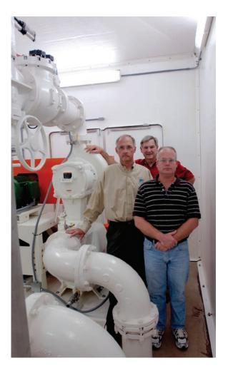
In this case, WCRSA utilizes a level control system into the pump's control panel. For communication requirements for that data, WCRSA relies on a RACO dialer, which is also used on all WCRSA pump stations for data monitoring.
