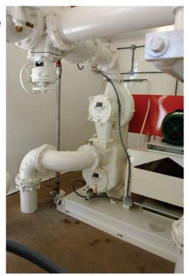
result. Because of the area served by the pumps, the station took into account a yield of 800 gallons per minute to achieve a total dynamic head of 160 feet. A conventional, single pump was incapable of delivering this type of volume and pressure. The plan was drafted to incorporate two T-series pumps, operating in a series, one right behind the other, in order to obtain the required head.
