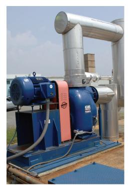
With traditional vertical-line sump pump designs, the pumps remain housed in tight, confined spaces. Therefore, when a team member needed to enter the area for maintenance, a series of confined space entry procedures had to be followed to secure personnel safety. Otherwise, an overhead crane was required to remove the pump from the area, which was a lengthy process – often an all-day procedure.
