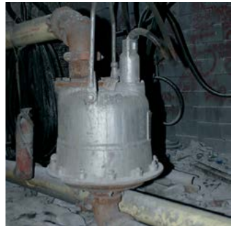
In-line staged submersible pump increases pumping distance.
