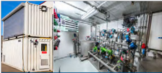
Packaged Chemical Additive Facilities
