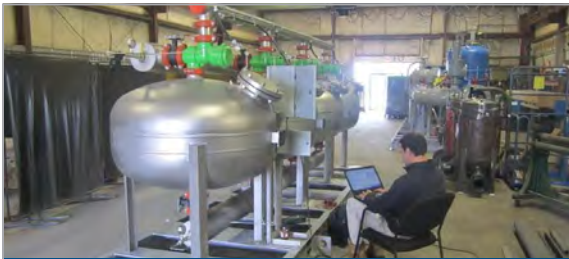
Gland Seal Filter Systems
