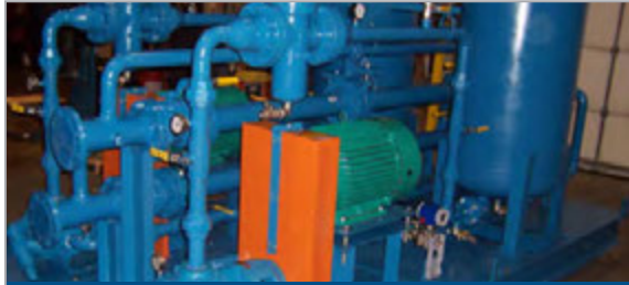
Diesel Fuel Pump & Coalescers Skids
