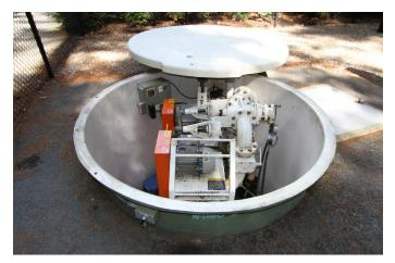
This below-ground lift station is one of the 27 stations in Raynham affected by nonwoven "flushable" wipes.
