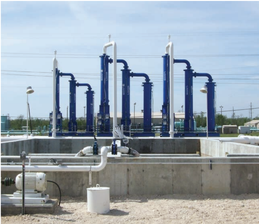
Above: Three (3) LAKOS Super Separators in series (JPX models) Below: Piping diagram and illustration of purge pit disposal area
