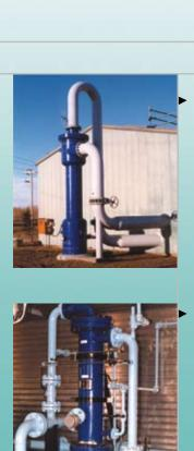
As primary filtration, a LAKOS Desander keeps sand & silt from river water out of a plant's piping system, reducing overall system maintenance and fouling.
