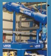
Sandy river water is pre-filtered with a LAKOS Desander to protect ultrafiltration equipment from excessive maintenance routines prior to high pressure injection wells.
