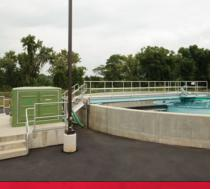
This ReliaSource® Above-Ground Submersible Valve Package (ASVP) utilizing SF Series® solidshandling submersible pumps transfers sludge at a wastewater treatment plant.
